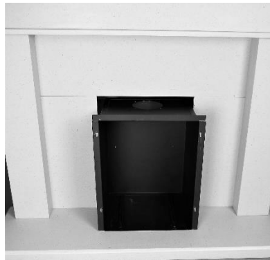
Fig J – Slide the convector casing into the pre-prepared fireplace (add additional insulation material above, sides and behind the convection case)
