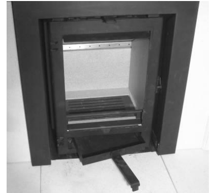
Fig K – Top air tubes must touch top of casing
